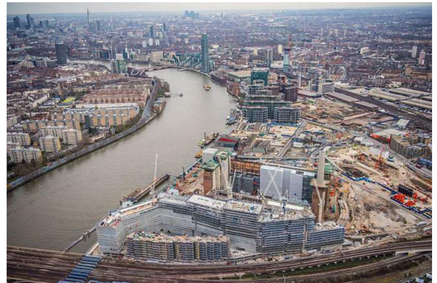
Aerial view looking east towards the City, showing the Nine Elms development area under construction (c.2016).
