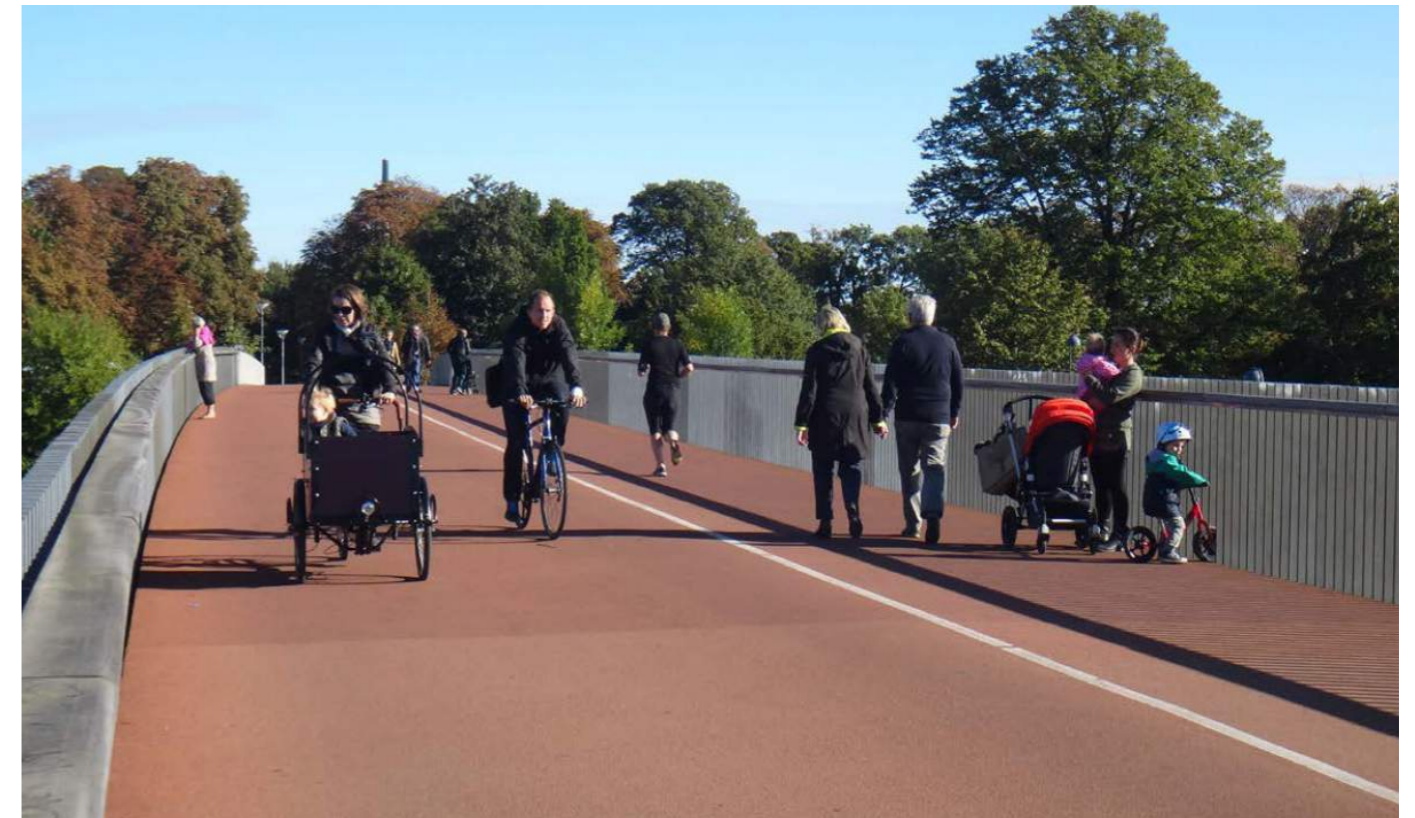
Pedestrians and Cyclists sharing a bridge in Copenhagen, Denmark
