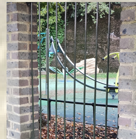
Railing panels in boundary wall
