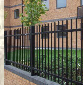
New panels on boundary wall
