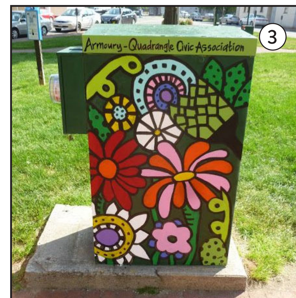
Existing Virgin Media Cabinet to be vinyl covered
