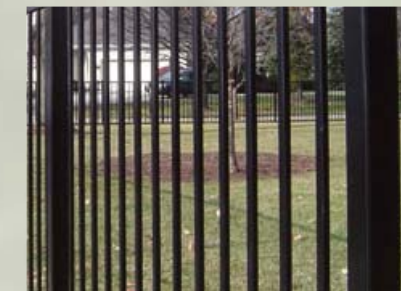
12. Railings refurbished and relocated
