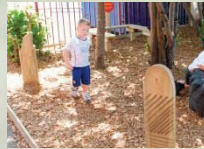
4. Loose bark mulch safety surface
