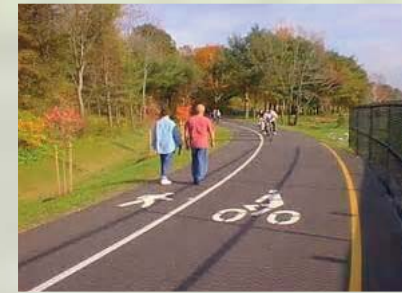
5. Cycle paths clearly designated using markings and/or coated tarmac in buff or green
