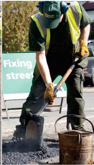
Repairing roads and pavements
