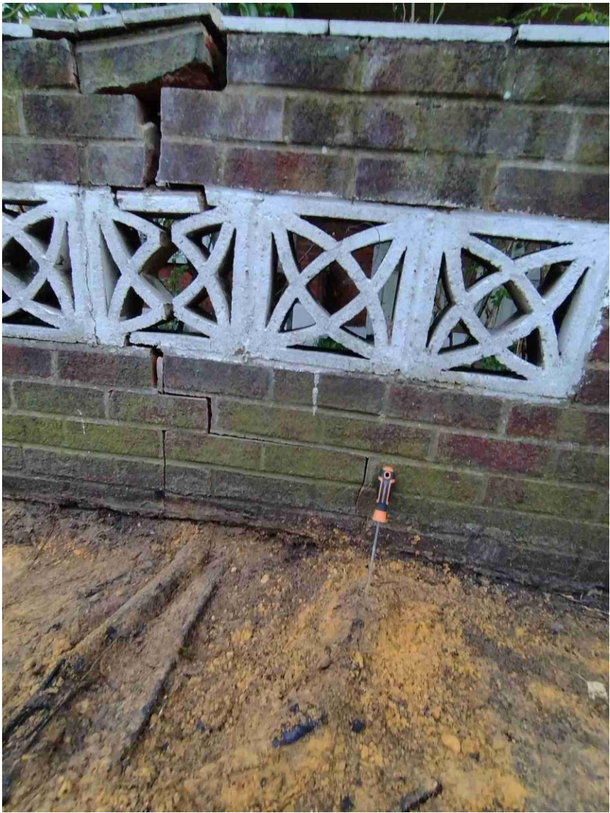
Image 3: Surface tree roots, wall & footway damage
