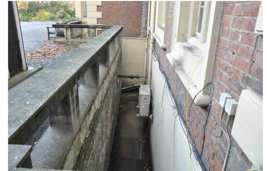
Figure 56: Blocked drainage network at northern lightwells
