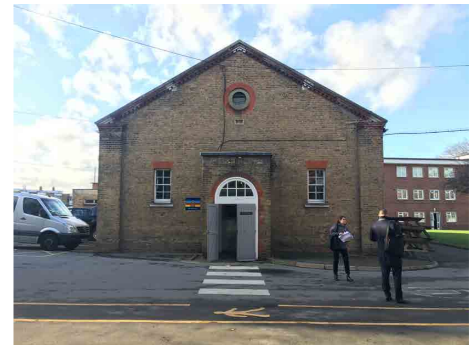
Figure 22: The former Band Practice Hall
