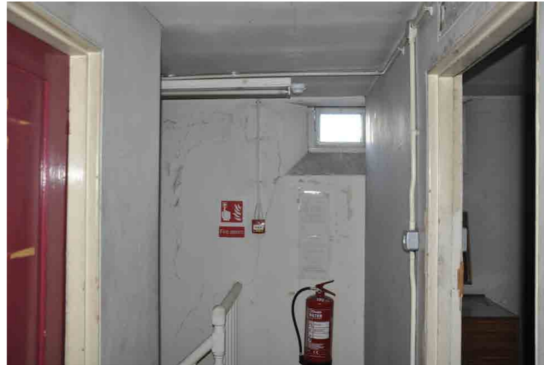
Figure 58: Signs of water ingress in the loft
