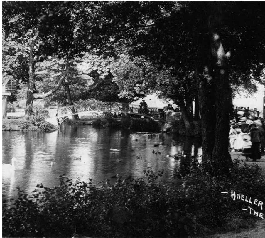
Figure 31: This 1907 photograph shows a bridge over the lake as described by the auctioneer in 1841
