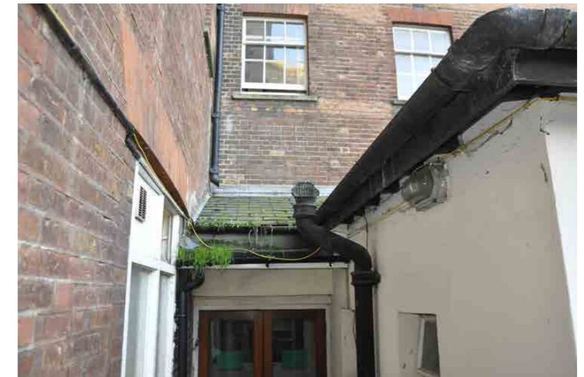
Figure 53: Blocked rainwater goods
