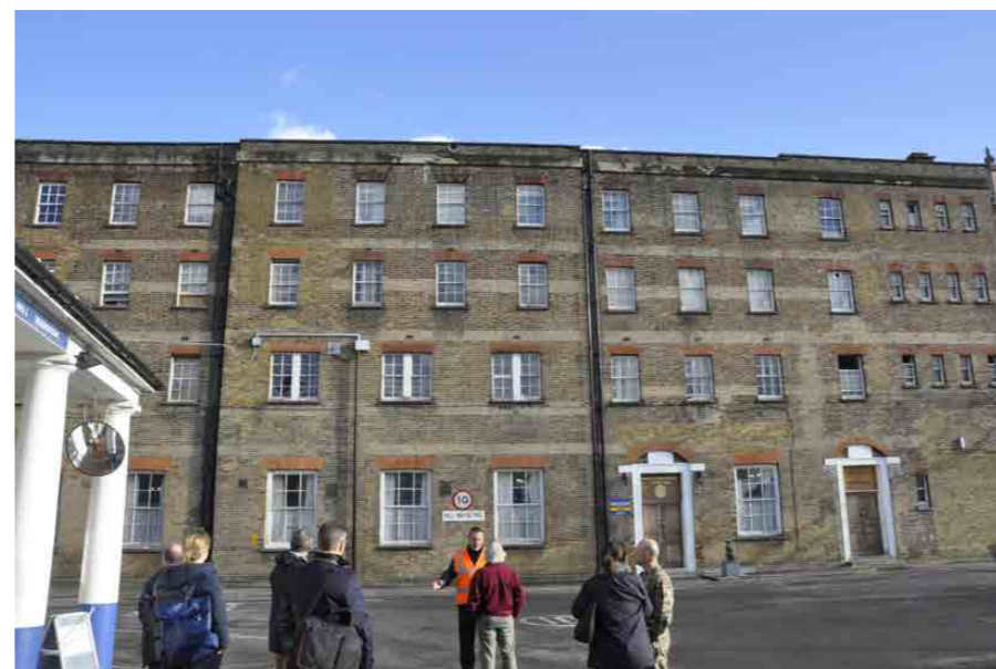
Figure 38: Western elevation of west wing
