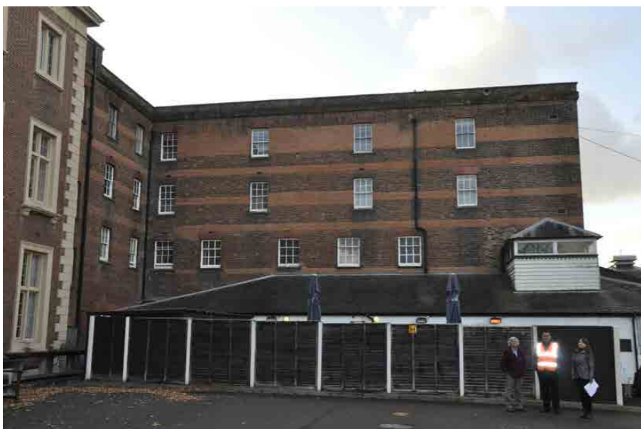
Figure 37: View of northwest wing from the east, showing the patched brickwork and the subsidiary building in front
