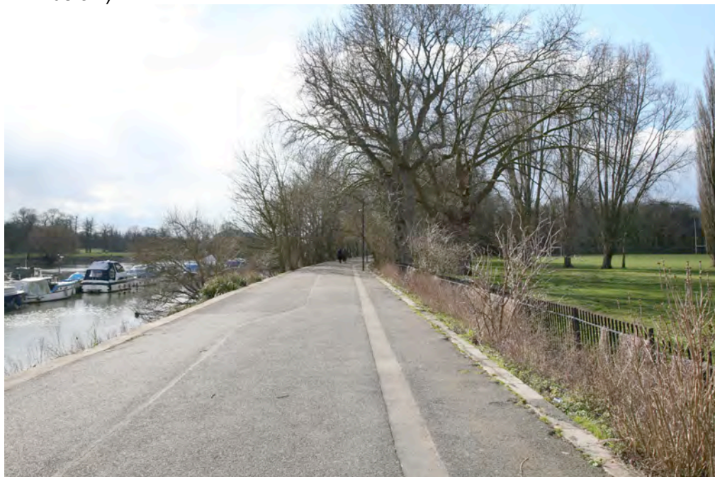
Figure 4.14 Pontoon moorings, flood defences and Marble Hill Park
