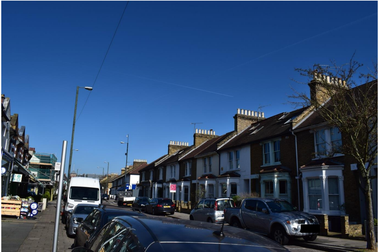
Housing along White Hart Lane East
