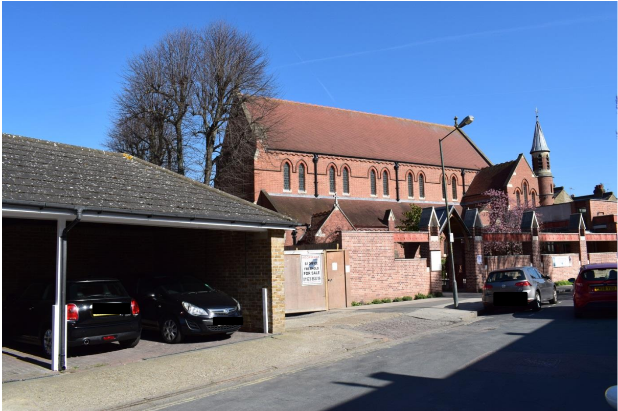
St Michael's Church and garages, Charles Street
