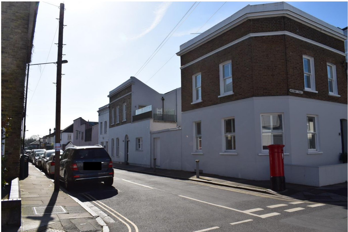
Cross Street Streetscene showing former public houses, and commercial buildings
