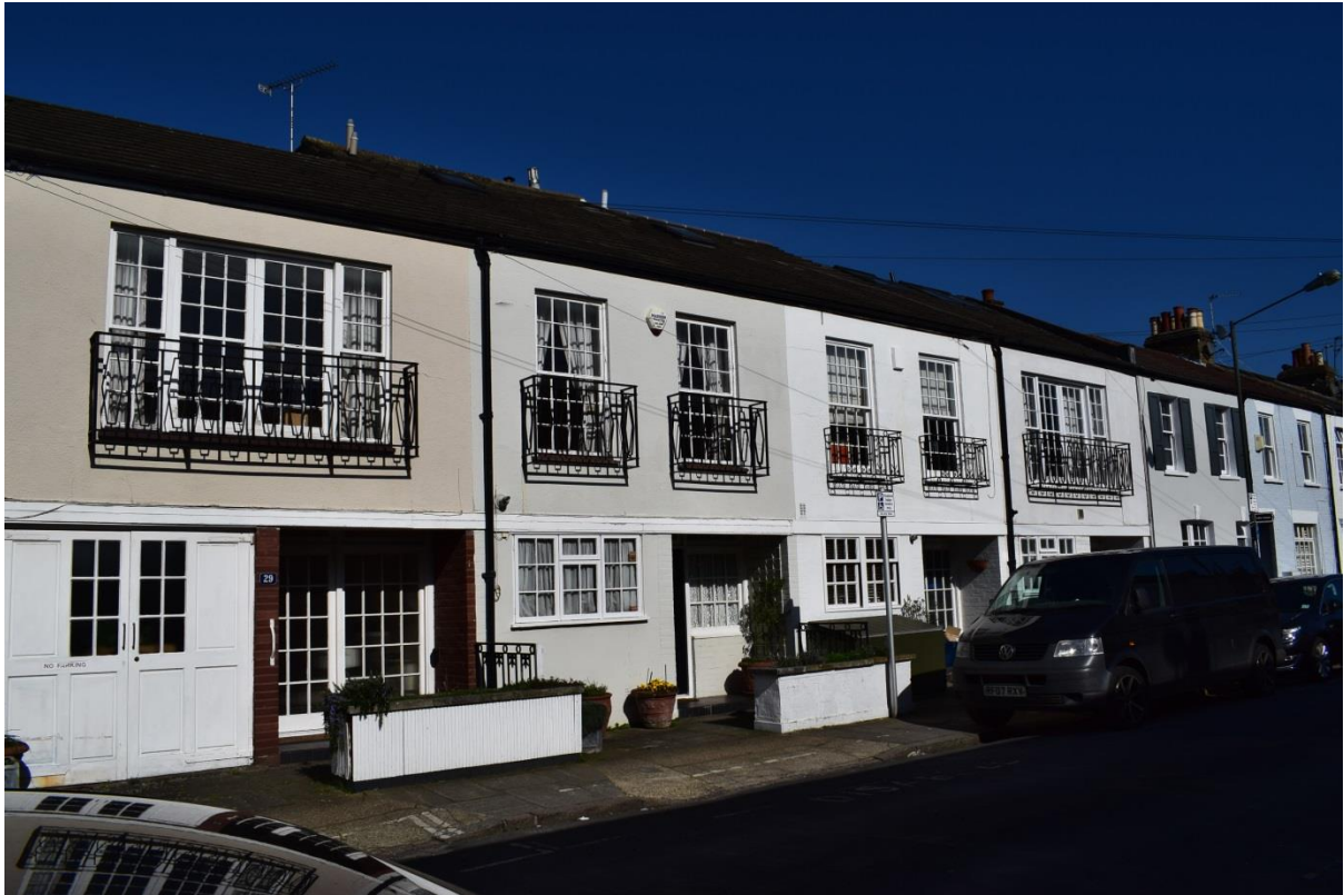
Juliet balconies installed along Westfields Avenue which is a negative influence to the streetscene
