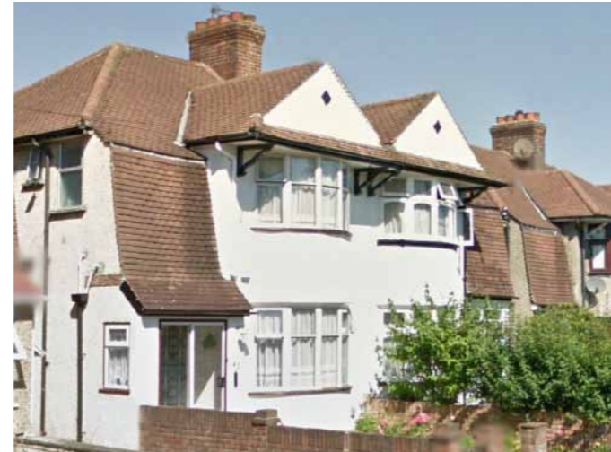
Arts and Crafts style, multiple pitched roofs, tile detail on a pitched gable, bow window. This pair of adjoining properties have white painted render
