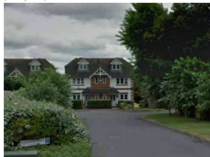
Use of red brick, render and symmetrical elements (Shelburne Drive)
