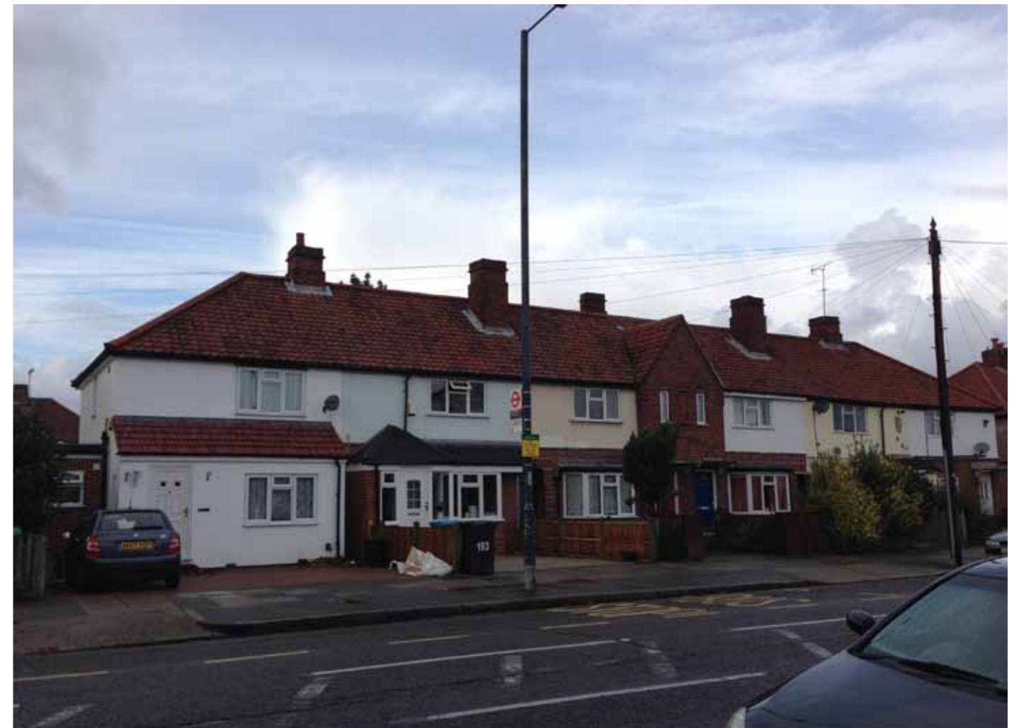
Hospital Bridge Road
