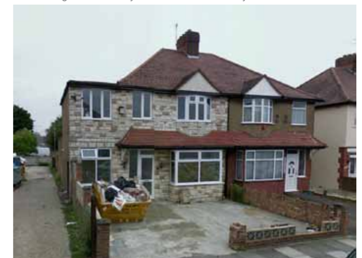
Chose replacement windows, soffits, barge boards, gutterings, roof tiles and doors that complement your house style. Think about mortar when re-pointing brick work.
