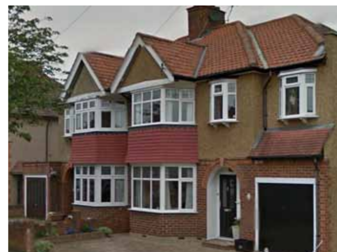
Red brick and pebbledash with red hung tiles on bay projections (this property is also a good example of a well integrated extension)
