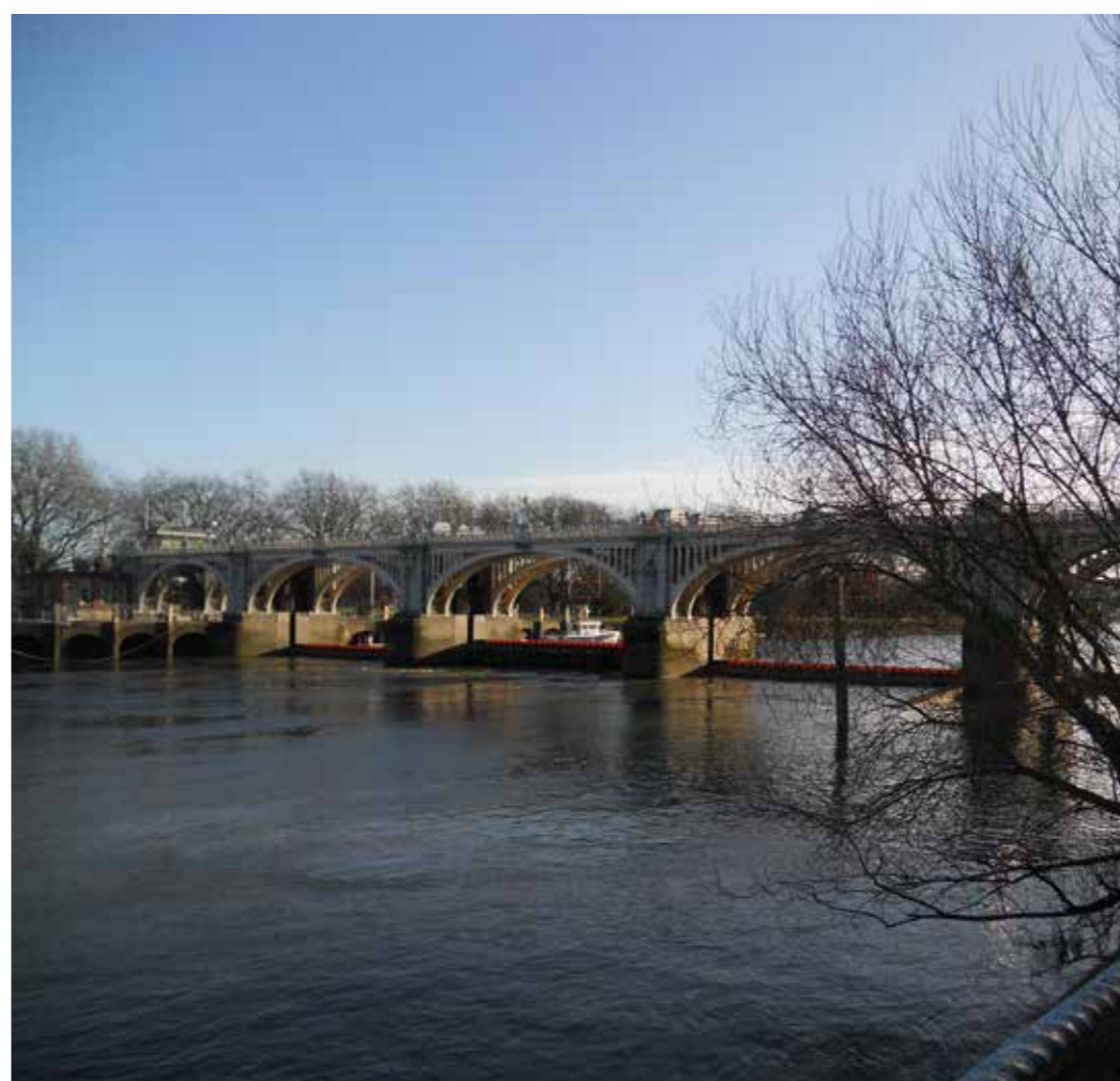
Richmond Lock Footbridge
