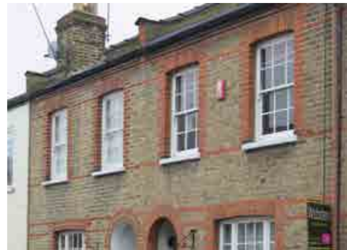
Traditional sash windows
