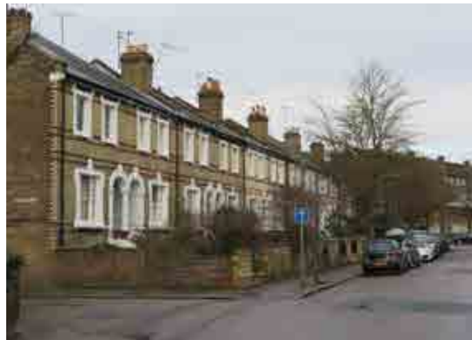
Terraced housing along Haggard Road
