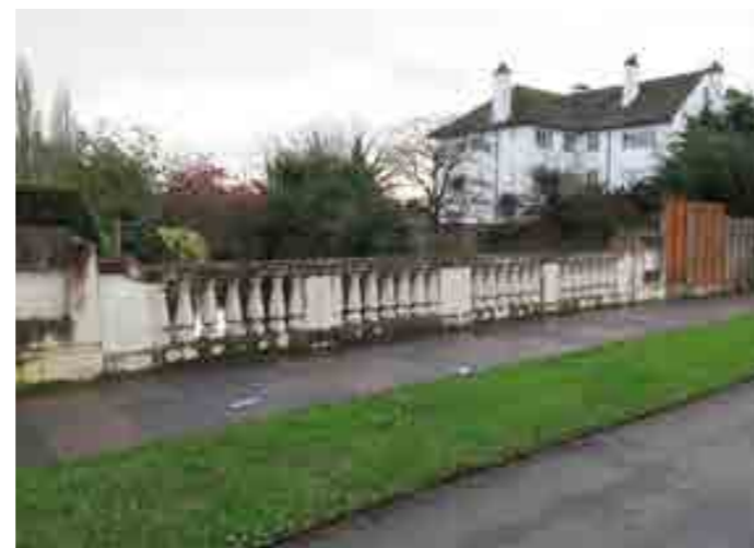
Chertsey Road bridge
