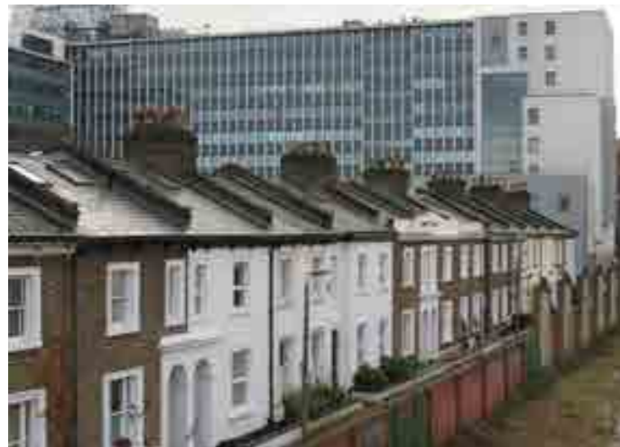
Mary's Terrace with modern development in the background
