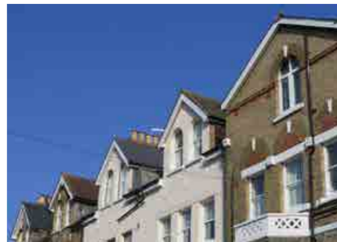
Gable roofing along the eastern side of Queen's Road
