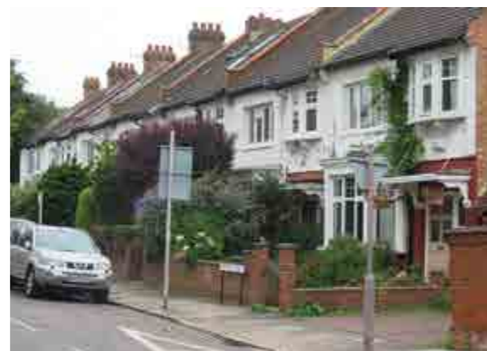
Radnor Road looking north
