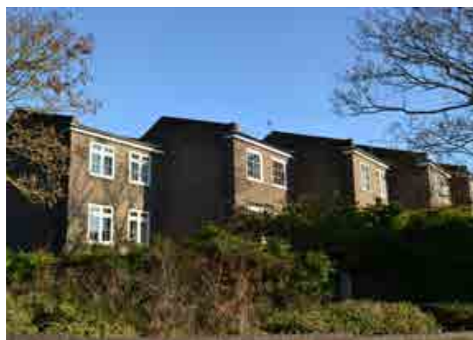
Back of Fortescue Park
