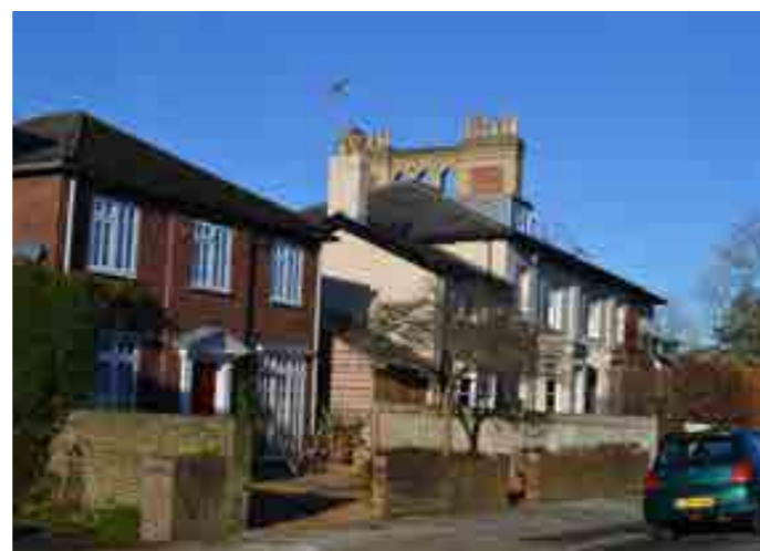
View north along Pope's Avenue
