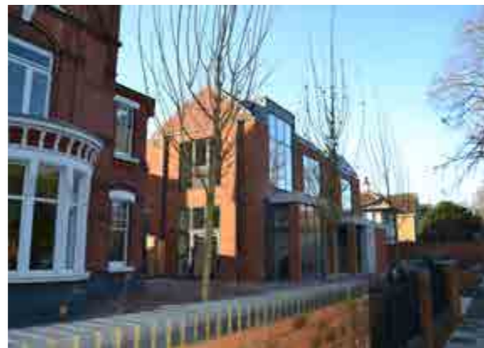
Newland House School
