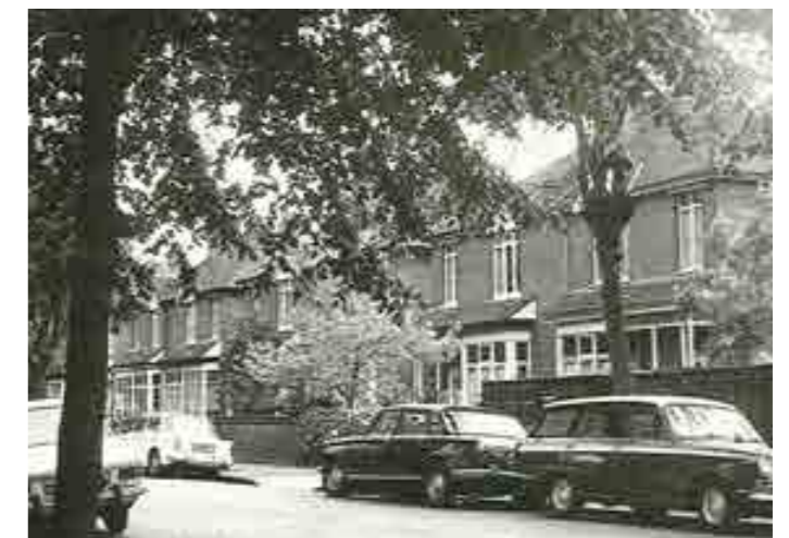
1973 photograph of 22-24 Walpole Road
