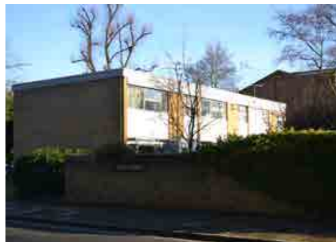
The houses are built of stock brick and have two-tone painted timber windows
