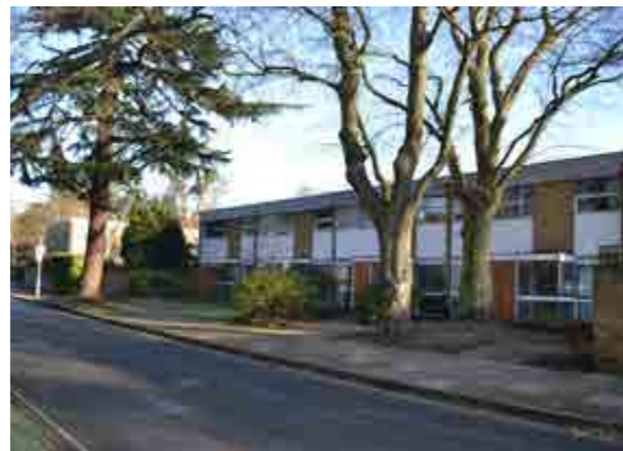
Two storey uniform terraced housing
