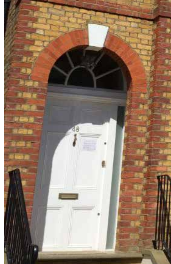
Panelled door with fanlight in a modern house
