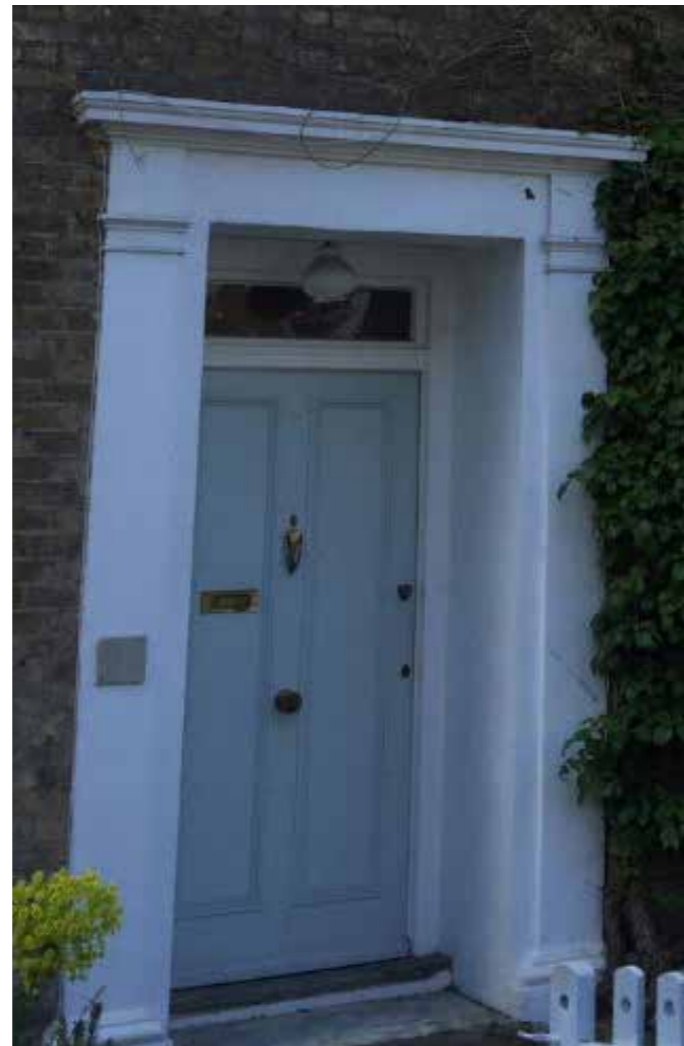
Two-panelled timber door with rectangular fanlight in a Victorian house
