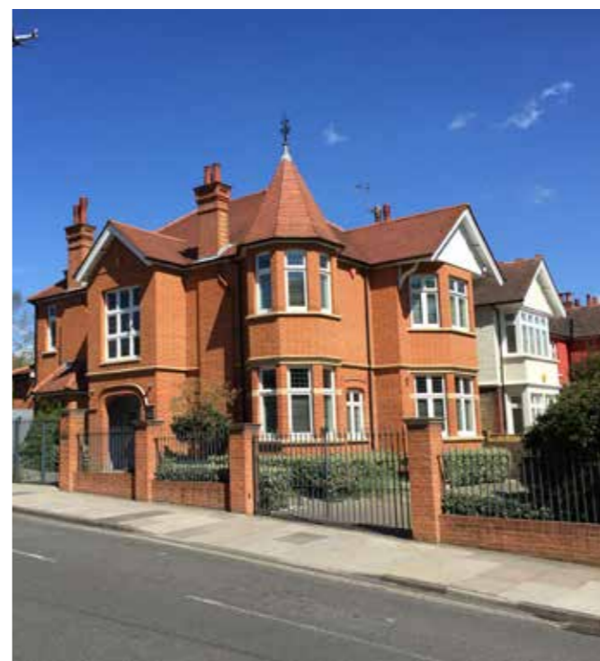
Iron railings, Queens Road
