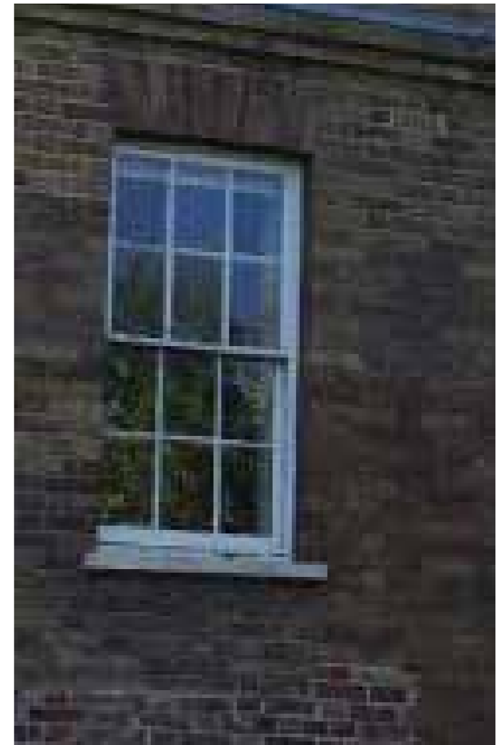
Six over six timber sash windows in a Georgian house
