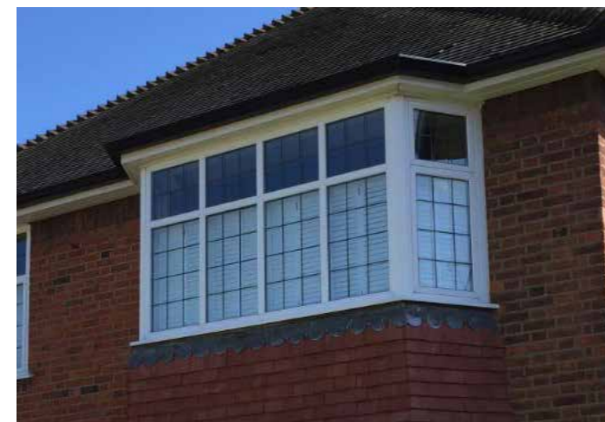
Timber casement windows with leaded lights in a twentieth century house
