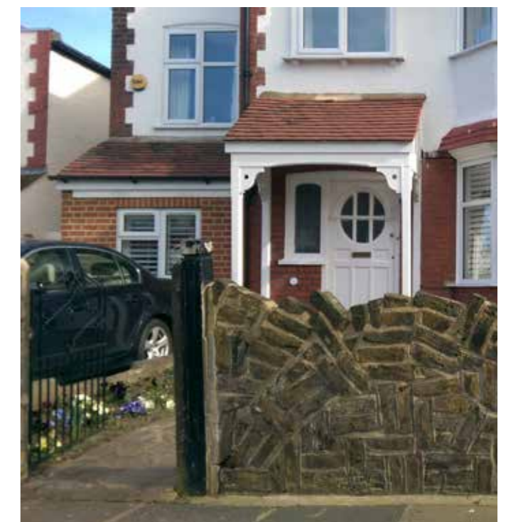
Boundary wall, Clydesdale Gardens
