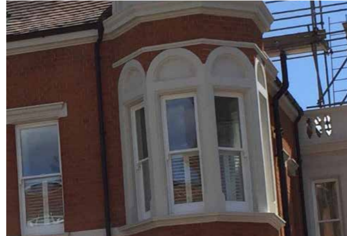
Timber sashes in a Victorian turret
