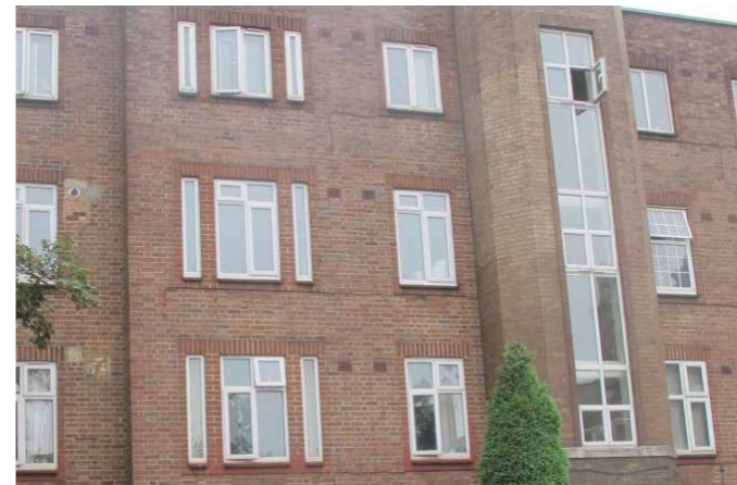
Art deco-influenced metal-framed windows with casement openings; many of those to the left and right have been replaced with uPVC window in differing styles, those at the highest level retaining the greatest sense of the original design
