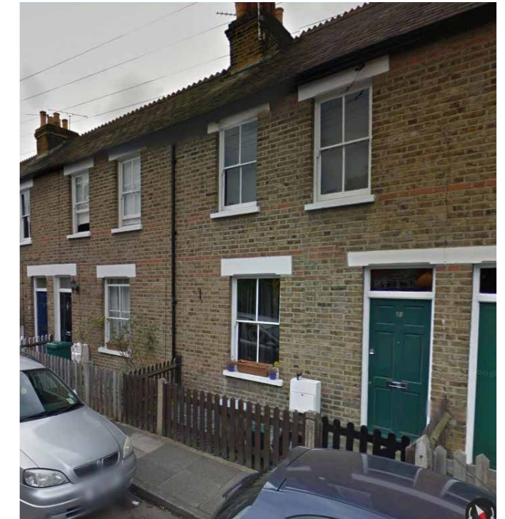
Fencing - Victoria Road
