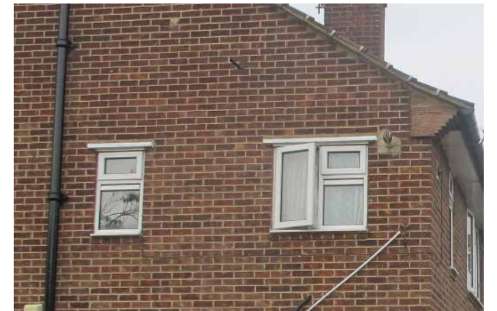
Post-war uPVC windows with different casement openings
