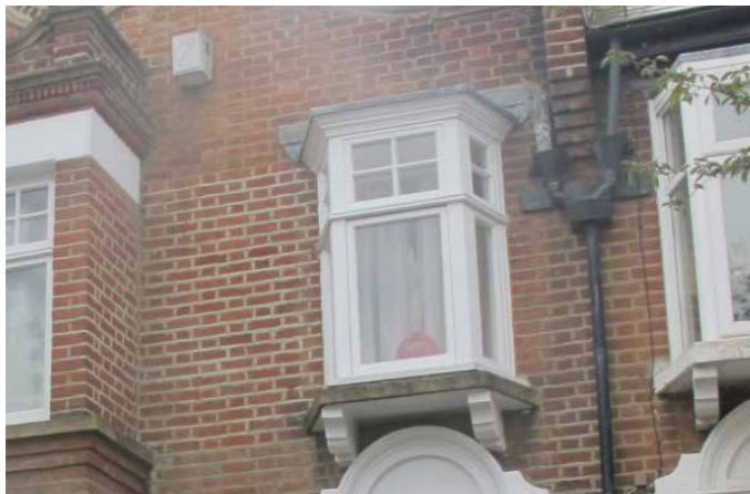
Edwardian timber oriel window with casement opening
