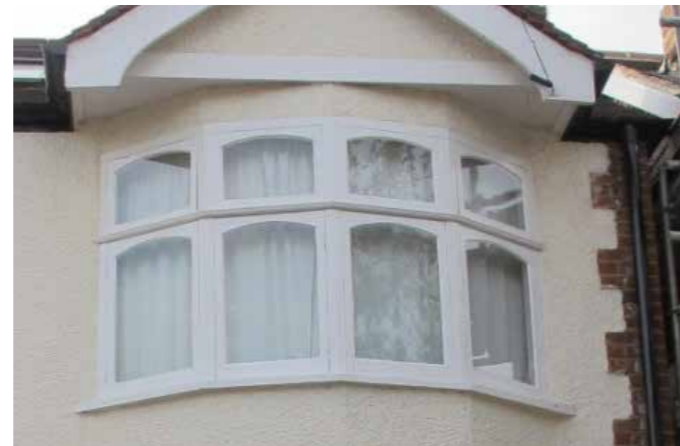
Inter-war timber bow window with casement openings and arched apertures
