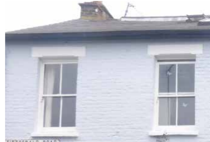
Victorian four-pane sash windows with flat artificial stone lintel
