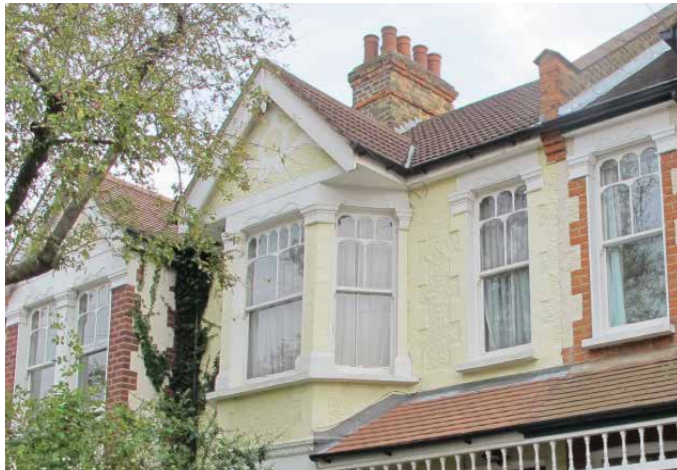
Late-Victorian hybrid sash windows in a canted bay with Classical-moulded reveals, the upper sash containing an arcade motif of shaped panes framed in fine timber girdles
