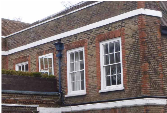
Georgian six-over-six sash windows, set flush with the façade in rectangular brick reveals
