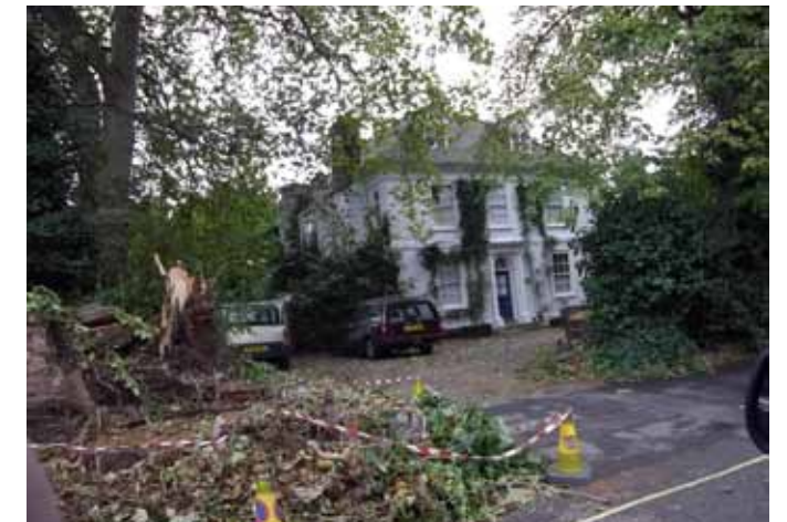
West Hall, West Hall Road
