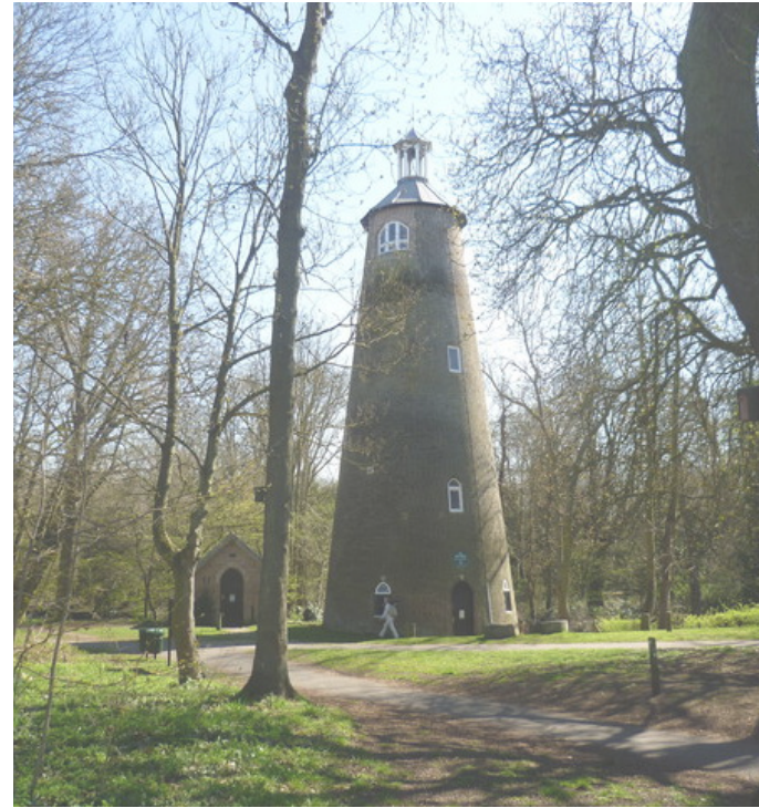
1 - The Shot Tower context in Crane Park amongst Willow and Alder trees
