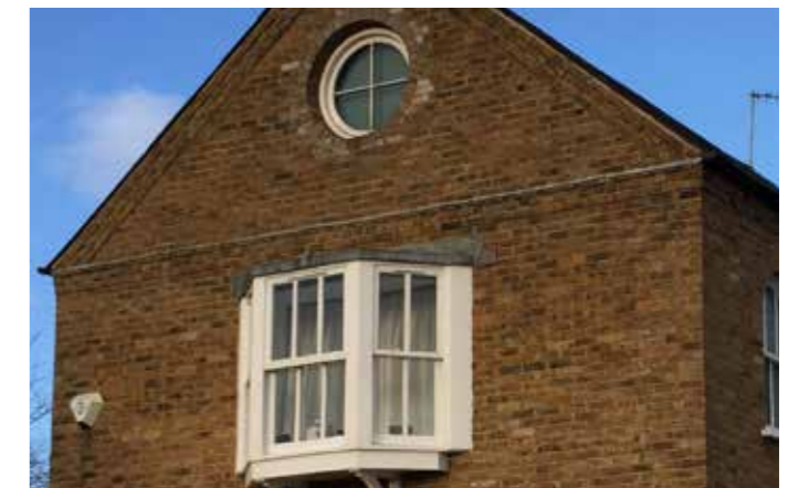
Timber Canted bay sashed window. with a circular porthole window above
