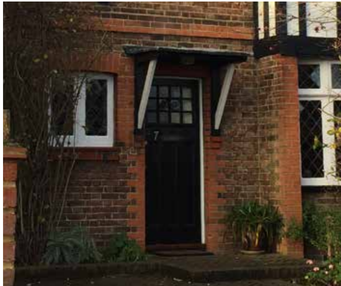
Timber casement doors with simple porch overhang
