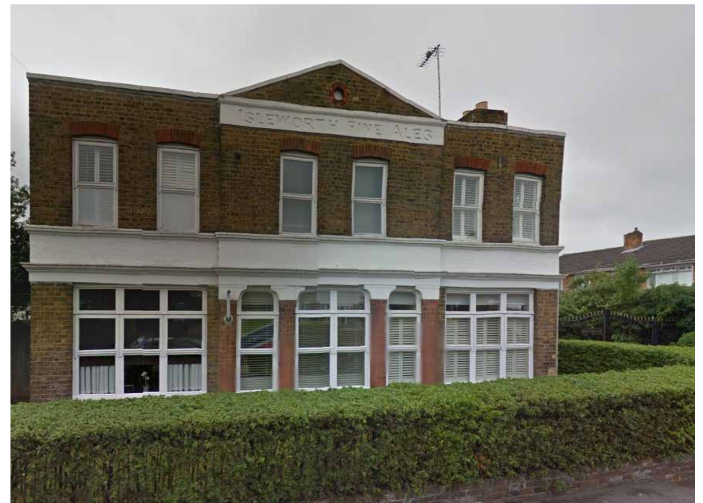
Former Public House, Uxbridge Road
