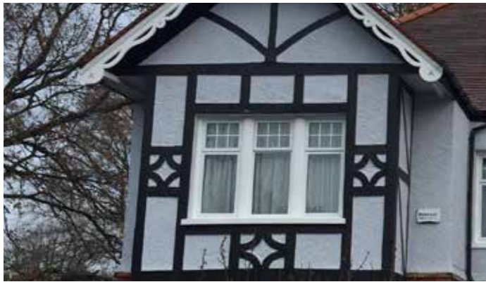
Painted render and timber frontage and timber casement windows
