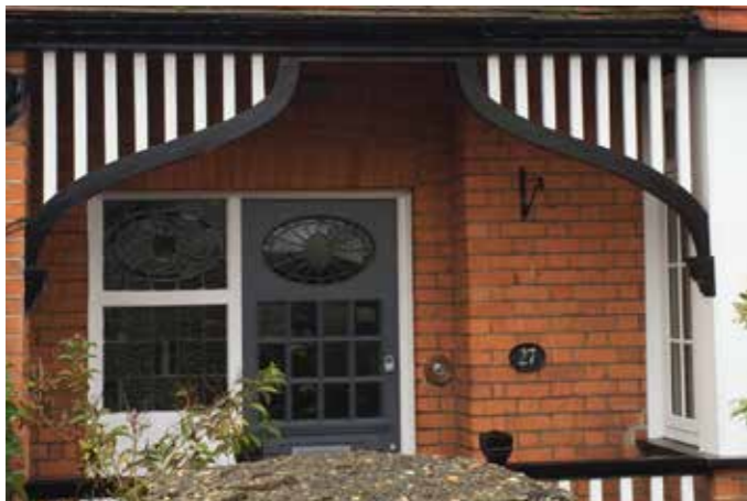
Timber front entrance door with oval stained glass glazing. Porch surround includes significant black and white painted timber consoles
