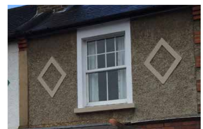
Half colonial sash window with original render detailing either side
