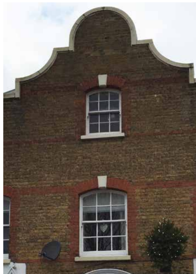
Dutch gabled frontage with stock brick, white painted keystones above six over six sash windows
