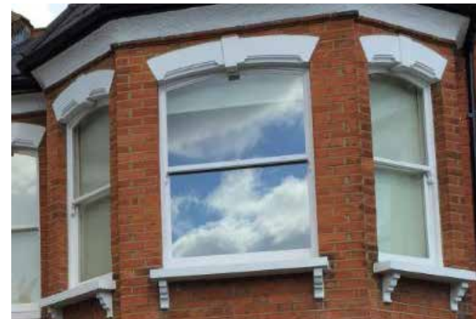
Timber sash window in a Victorian house
