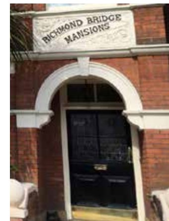
Timber panelled door in a c. 1900 mansion block
