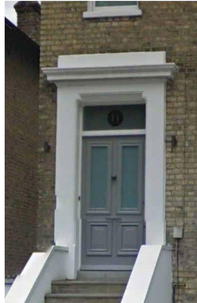
Timber panelled double doors in a Victorian house
