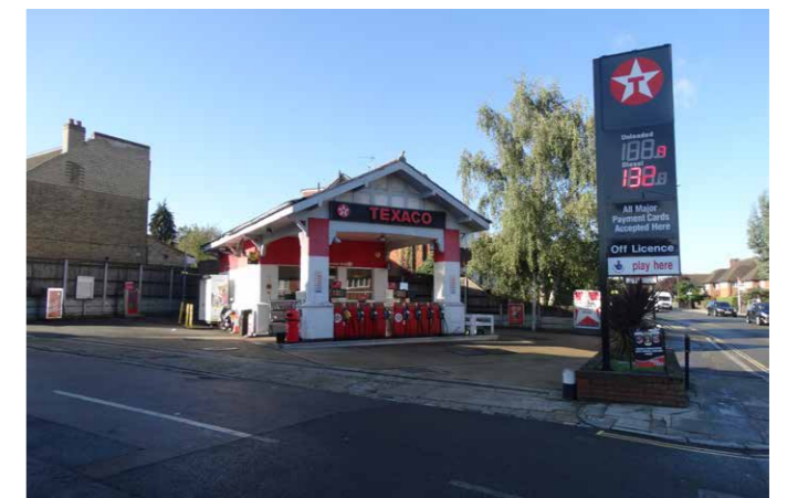
Grade II listed petrol station, Upper Richmond Road West
