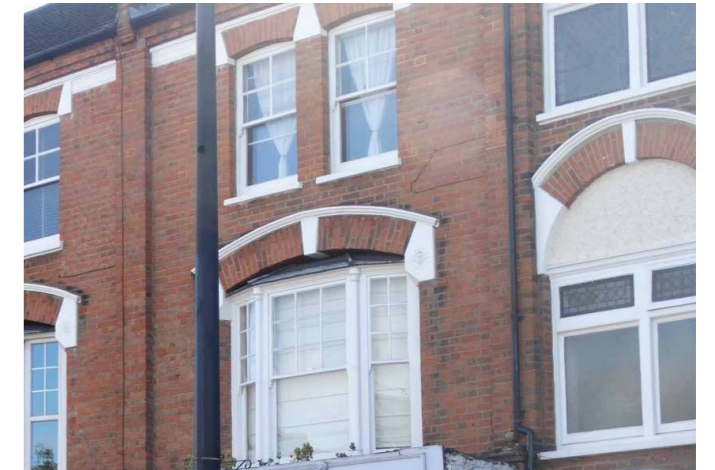
Edwardian hybrid sash windows, set in a timber gently-projecting canted bay within a three-centred arch reveal with decorative detailing
