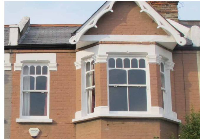
Edwardian hybrid sash window in projecting canted bay, with arched apertures in the upper sash
