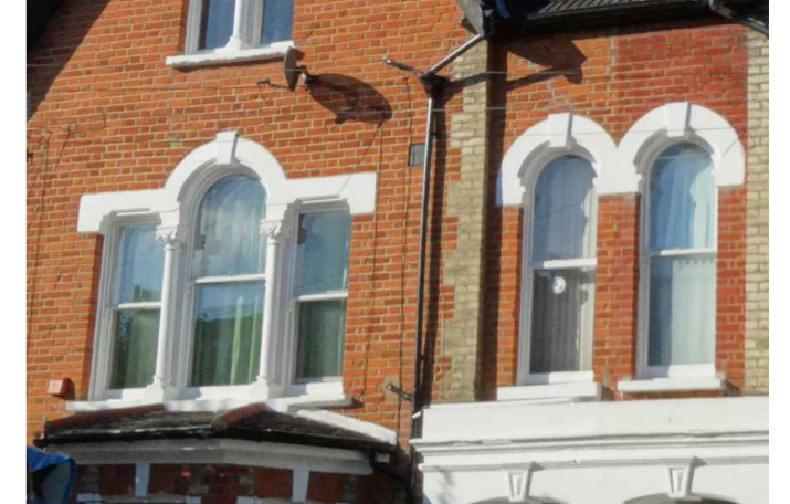
Victorian Classical sash windows with arched upper sash and decorative plasterwork column jambs
