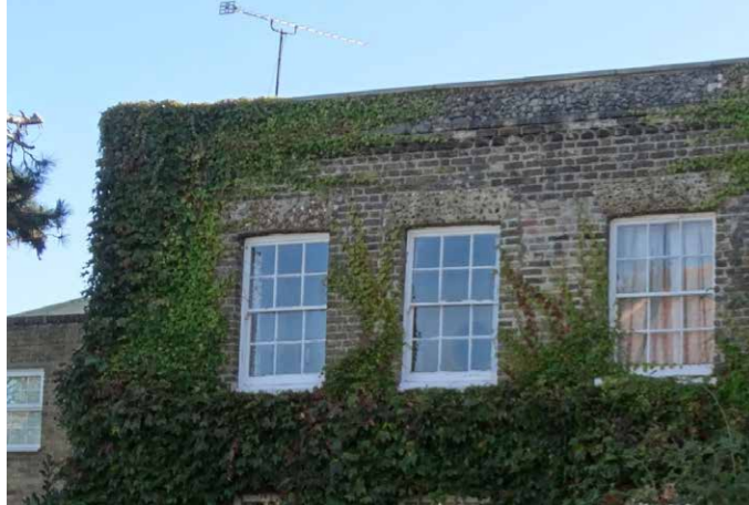
Georgian-style six-over-six sash windows, here featuring 'horns' typical of later sash window styles
