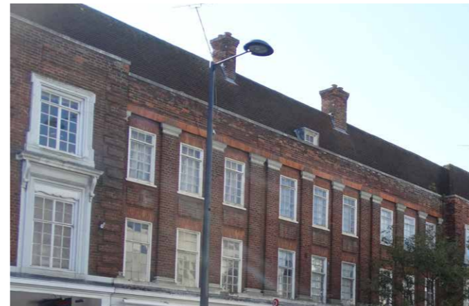
Interwar neo-Classical metal-framed windows
