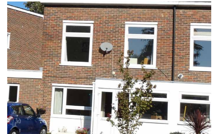
Post-war uPVC windows: with high transom (above) and picture window-form (below)
