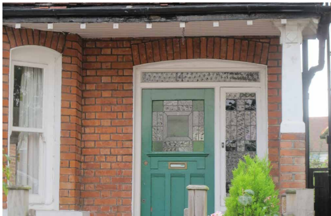
Edwardian narrow sash in a canted bay and, around the door, leaded stained- and textured-glass side light and transom light
