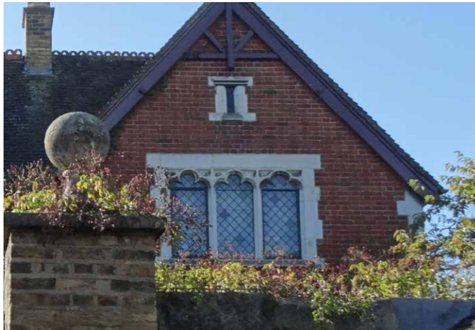
Victorian Gothic revival trefoil windows in a stone reveal with leaded casements
