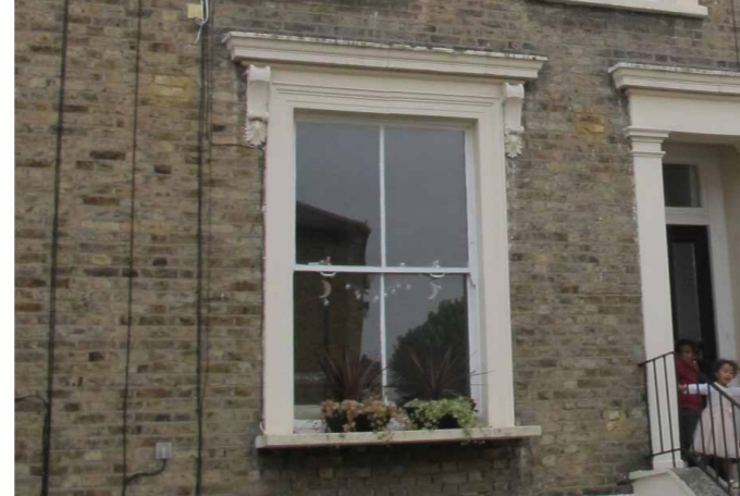
Victorian four-pane sash window
