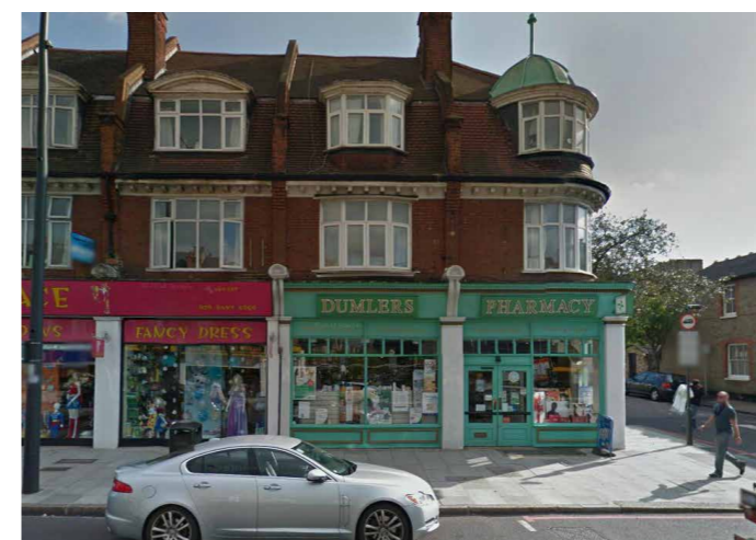
No. 495-497 Upper Richmond Road West
