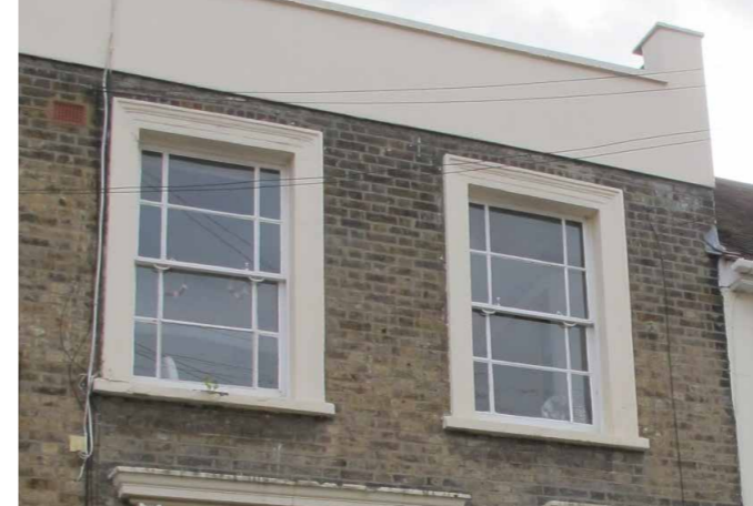
Victorian sash window with narrow-grille featuring margin lights
