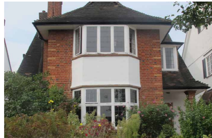
Edwardian Arts and Crafts-style leaded casement windows in the timber-frames of a projecting canted bay, under a low eave
