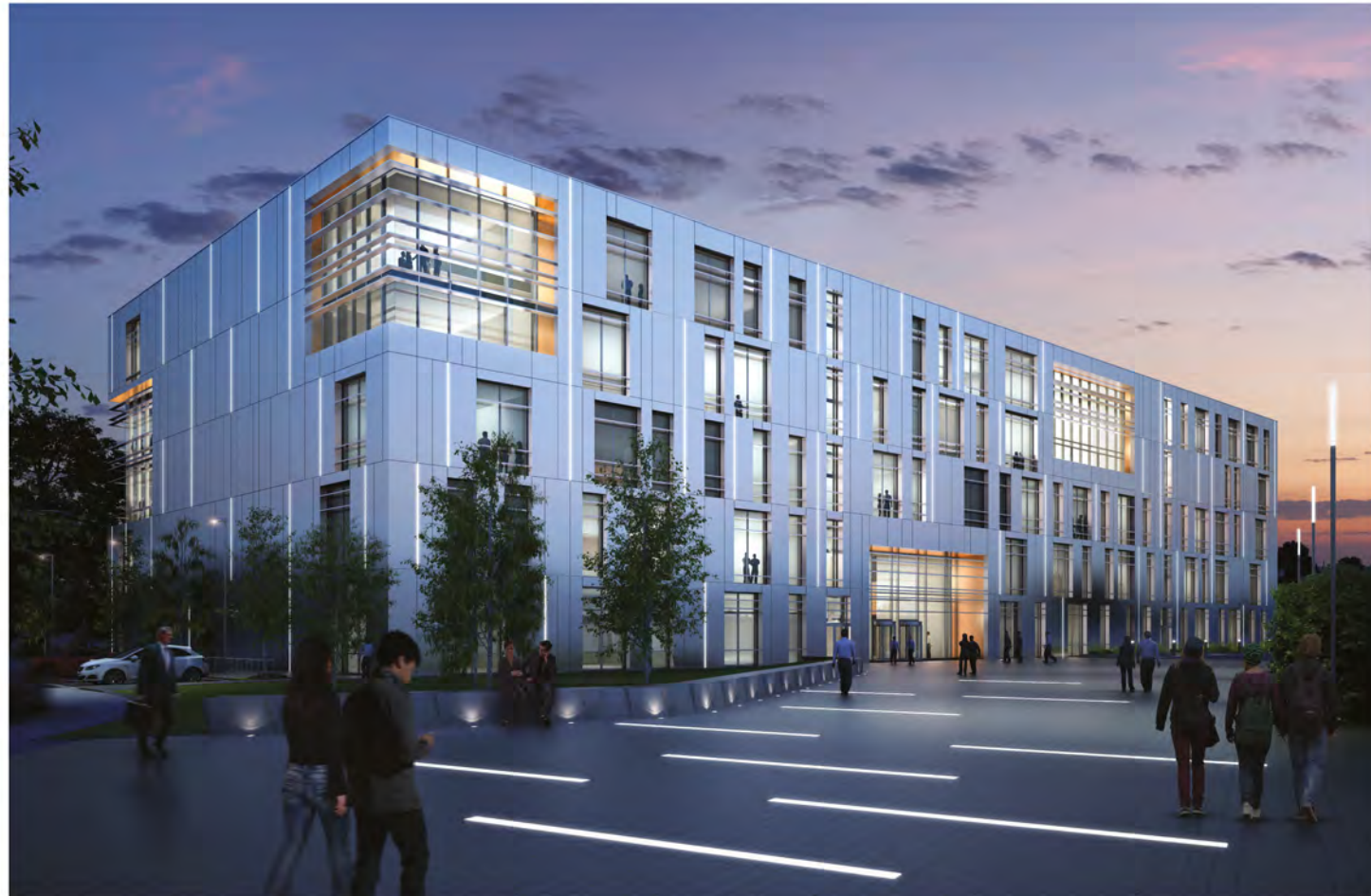
Looking across plaza towards main pupil entrance at dusk
