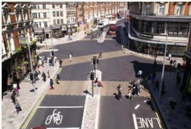
Crossing resurfaced with aggregate topping
