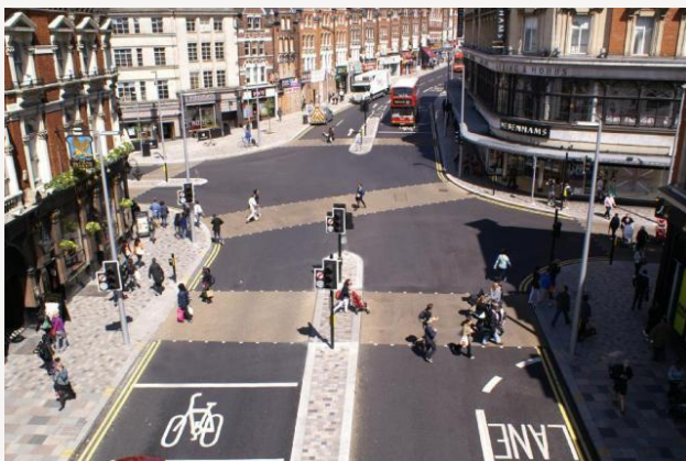
Crossing resurfaced with aggregate topping
