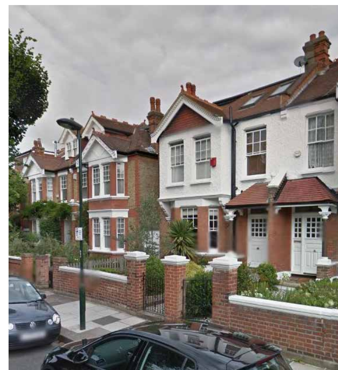
White capped walls and pillars - Westmoreland Road
