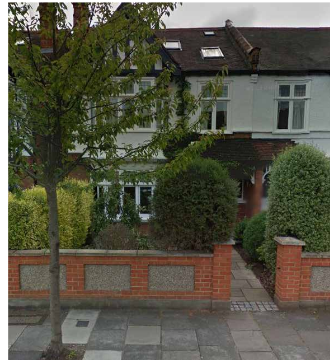
Boundary wall - Madrid Road
