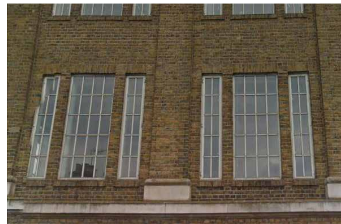
Interwar Crittall-style steel framed windows with casement openings
