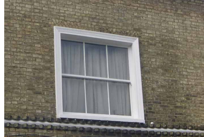
A Victorian three-light sash
