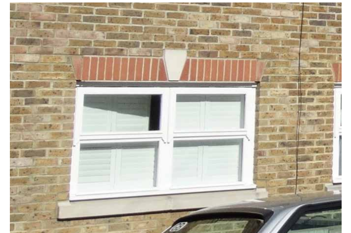
Late twentieth-century uPVC imitation sash window with horns
