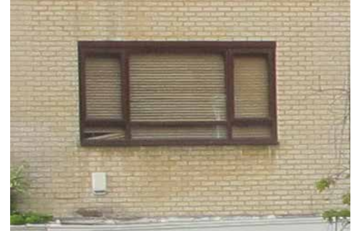
A twentieth-century uPVC picture window with side casements
