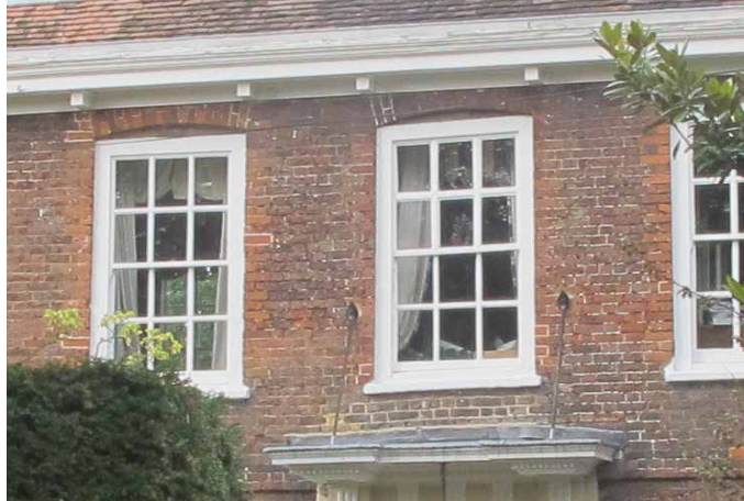
Georgian 'six over six' flush sash window
