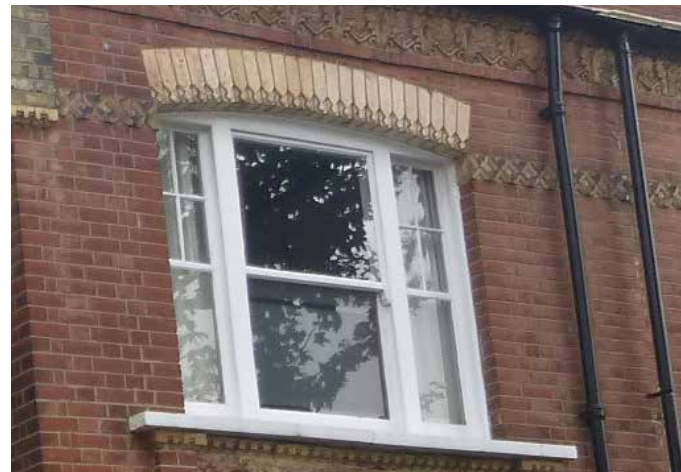
A tripartite late-Victorian or Edwardian window with central sash and hybrid margin lights
