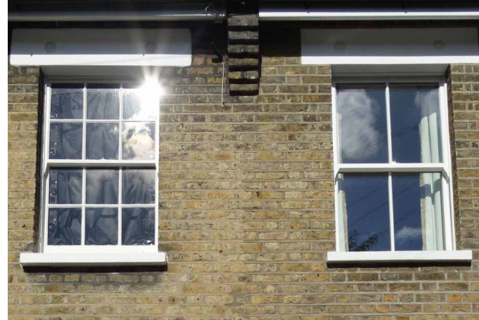
Georgian-style 'six over six' and two-pane sashes in the same Victorian terrace; both windows have typically Victorian 'horns' at the bottom of the upper sash
